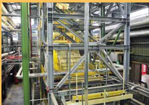
Steel structure for the forming line
